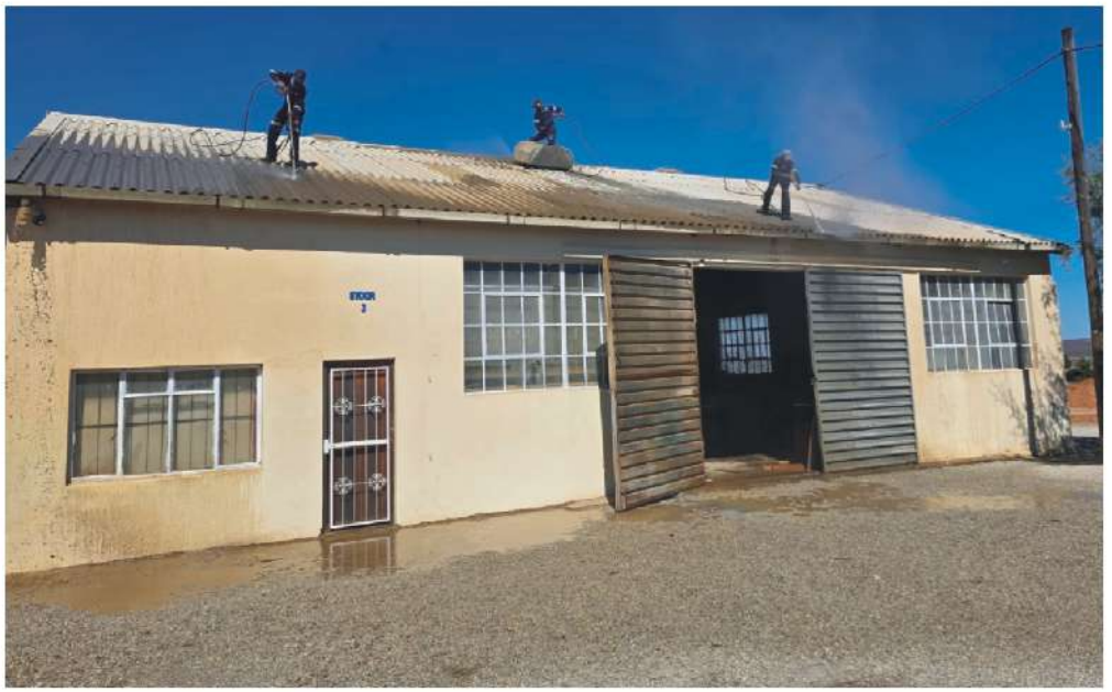
Workers busy cleaning a warehouse roof.
